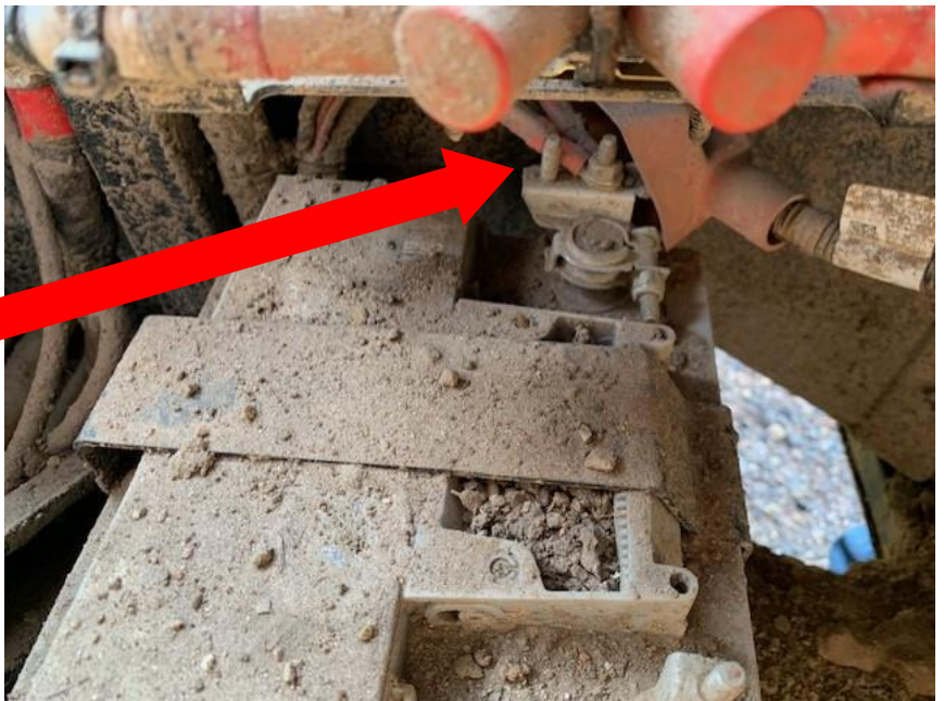
Battery Terminal Positive Stud
