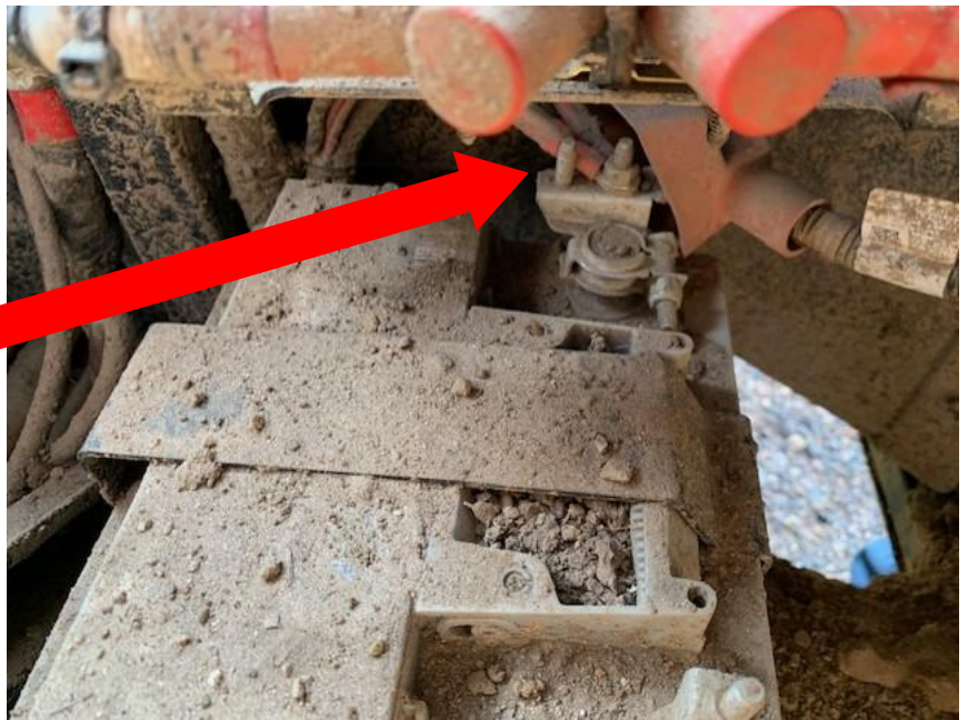
Battery Terminal Positive Stud
