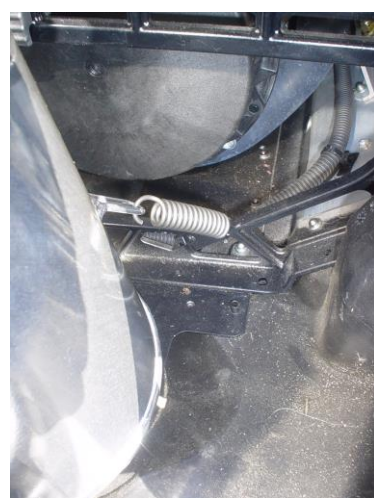
Front Lower Spring Installed #3
